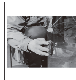
12.1 Install the hinge into the holes on the right glass.
