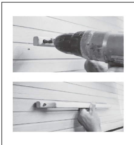
19. Install the towel rack (part J) with ST3.5*25mm screws (2 pcs).
