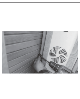
9. Install the beauty light (part P) using ST3.5*30mm screws (4 pcs).
